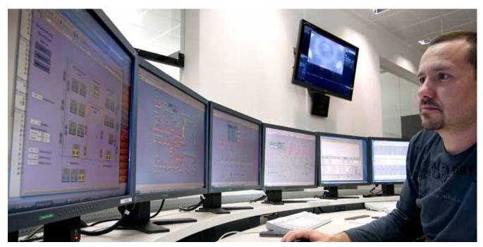
All eight workspaces in the areas of medium-voltage (six workspaces) and high-voltage (two workspaces) are each equipped with six monitors and thus ensure an optimum overview of all data and processes. User-friendliness is also considered: all six monitors can be operated with a single mouse, which also increases working efficiency considerably.
