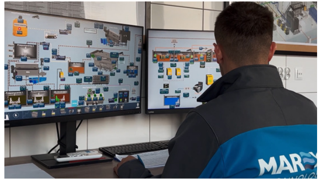
Control room overview of the wastewater treatment process
